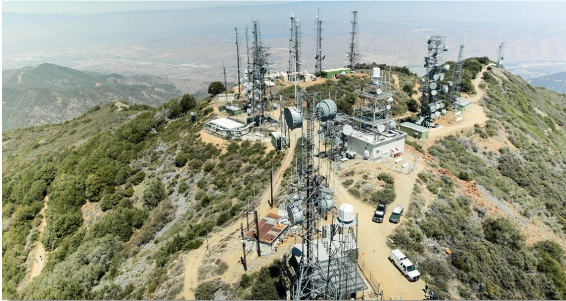
Figure 6 New Cameras Installed on SCE Telecom Tower in Orange County to Monitor Wildfire Activity May 9, 2018
